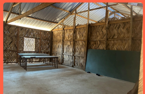
Newly constructed classrooms of Kumonggrikani St. Joseph School Chiringgro, William Nagar, Meghalaya
