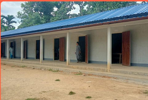
Newly constructed building of St. Mary's English School, Dholmara, Kokrajhar
