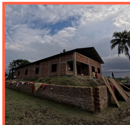
Under Construction Flood Shelter at Kathoni, Lahorighat, Morigaon
