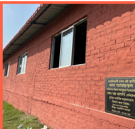
Flood Shelter at Boralimari, Hoiborgaon, Morigaon
