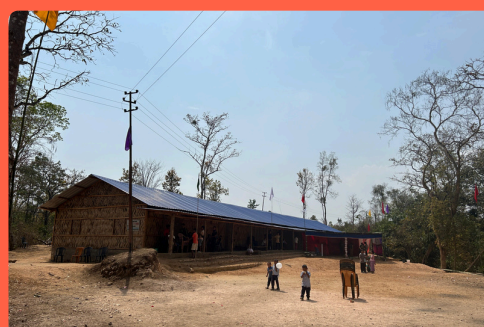
Newly constructed building of Kumonggrikani St. Joseph School Chiringgro, William Nagar, Meghalaya
