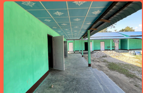
Corridor of the Nagapur School
