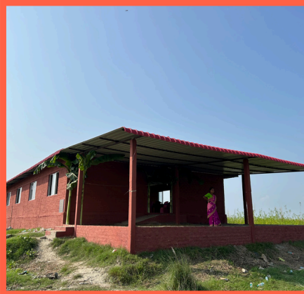
Flood Shelter at Boralimari, Hoiborgaon, Morigaon
