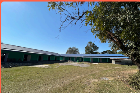
Newly constructed school buildings of Asha Darshan Nagapur School
