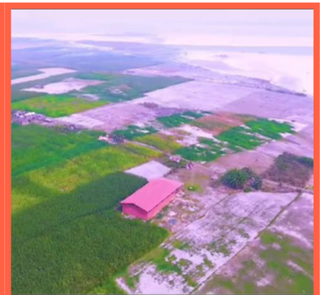
Bird's Eye View of the Flood Shelter at Boralimari
