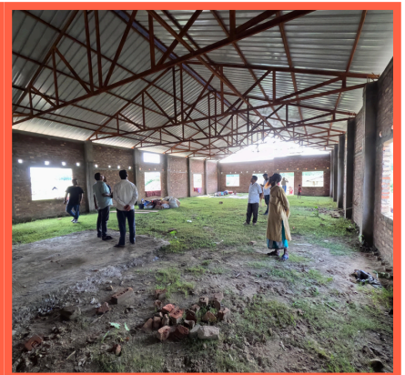
Under Construction Flood Shelter at Kathoni, Lahorighat, Morigaon
