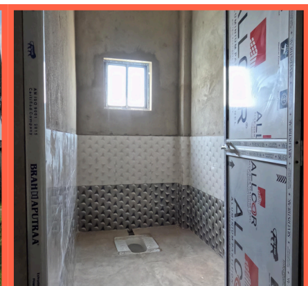
Toilet at the Flood Shelter at Kathoni
