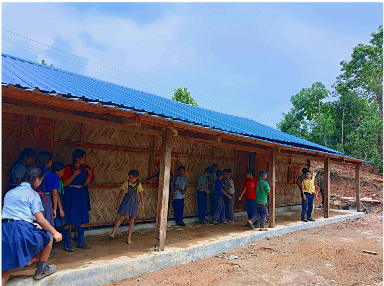
Newly Extended Classrooms at Ku-mongrikani St. Joseph School
