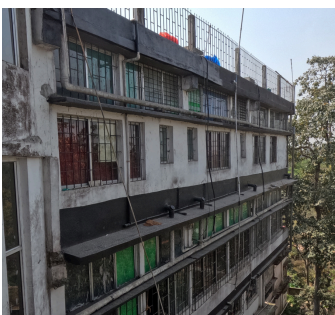
Waterproofing work at the Cachar Cancer Hospital
